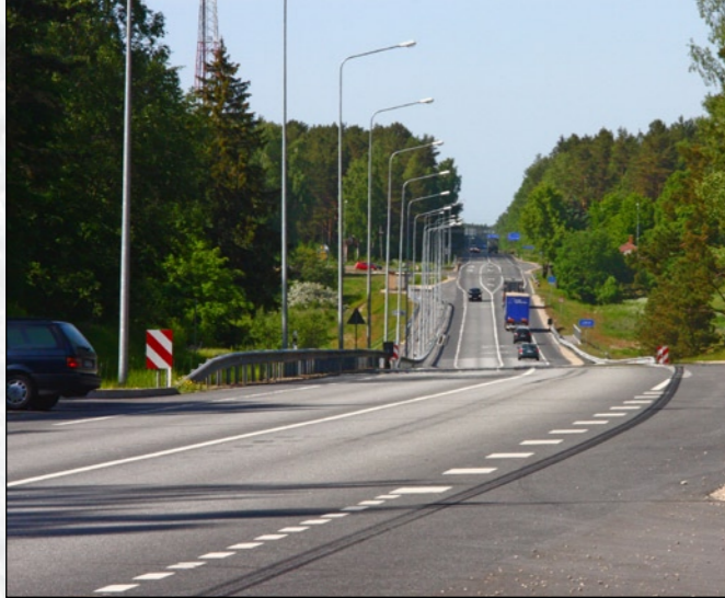
Reconstruction of highway "Via Baltica", 2007. Road section Skulte-Svētciems. Total km reconstructed — 40 km. Contracting Authority — Ministry of Transport
